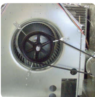
PowerMax DriveN Pulley on a Centrifugal Fan.
